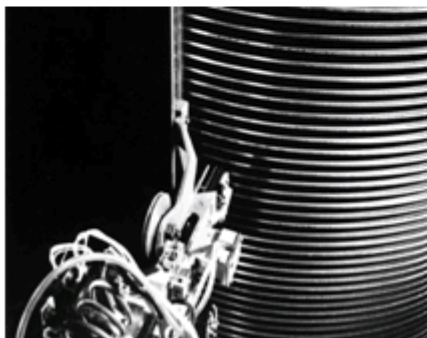
Sept. 13, 1956 – RAMAC – first hard drive shipped with 5 MB on 50 24" diameter disks
